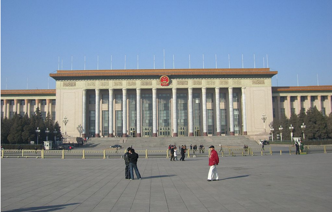
Figure 2. The Great Hall of the People on Tiananmen Square; note the classical columns and massing (Source: Delso, 2006).
