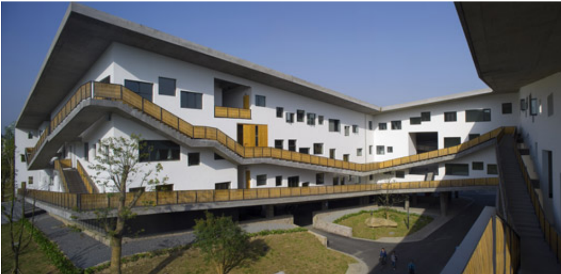
Figure 8. The Xiangshan Campus of the China Academy of Art in Hangzhou, designed by Wang Shu (Source: The Hyatt Foundation, 2017).
